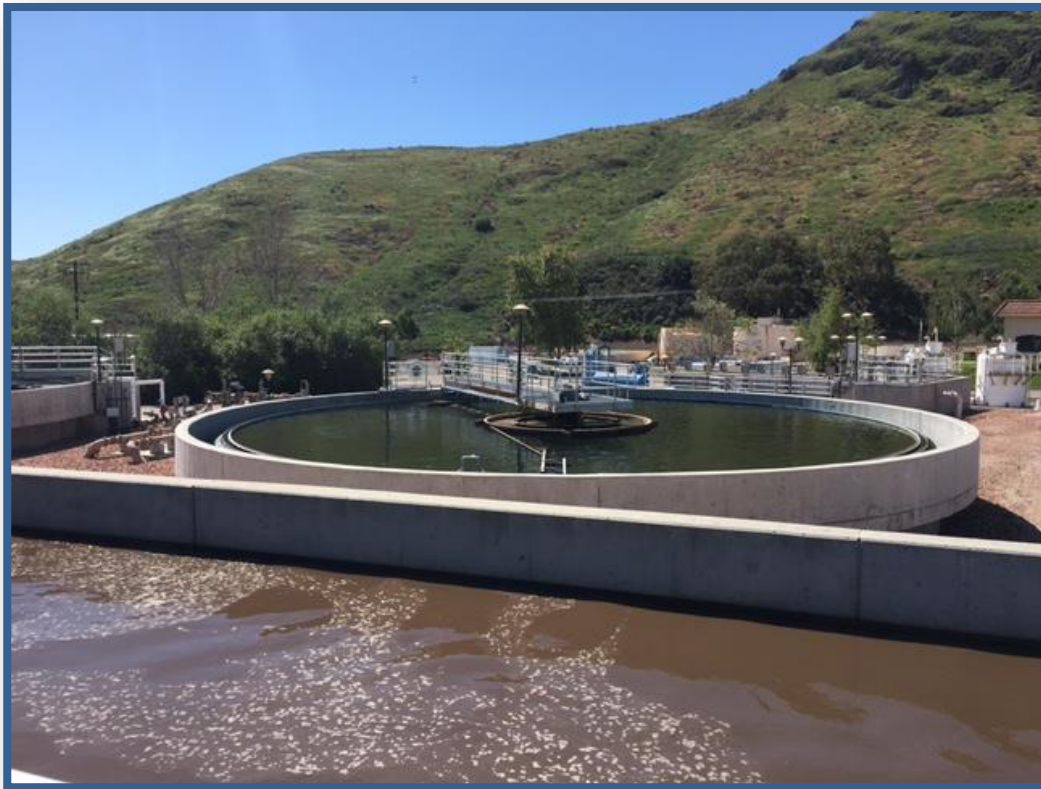
Camrosa Water Reclamation Facility, Secondary Clarifier
