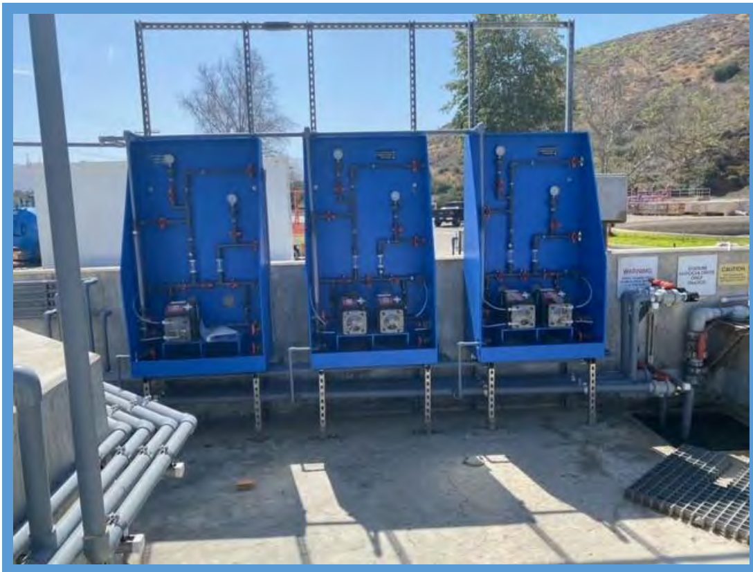
CWRF Chemical Tank and Feeder System upgrades
