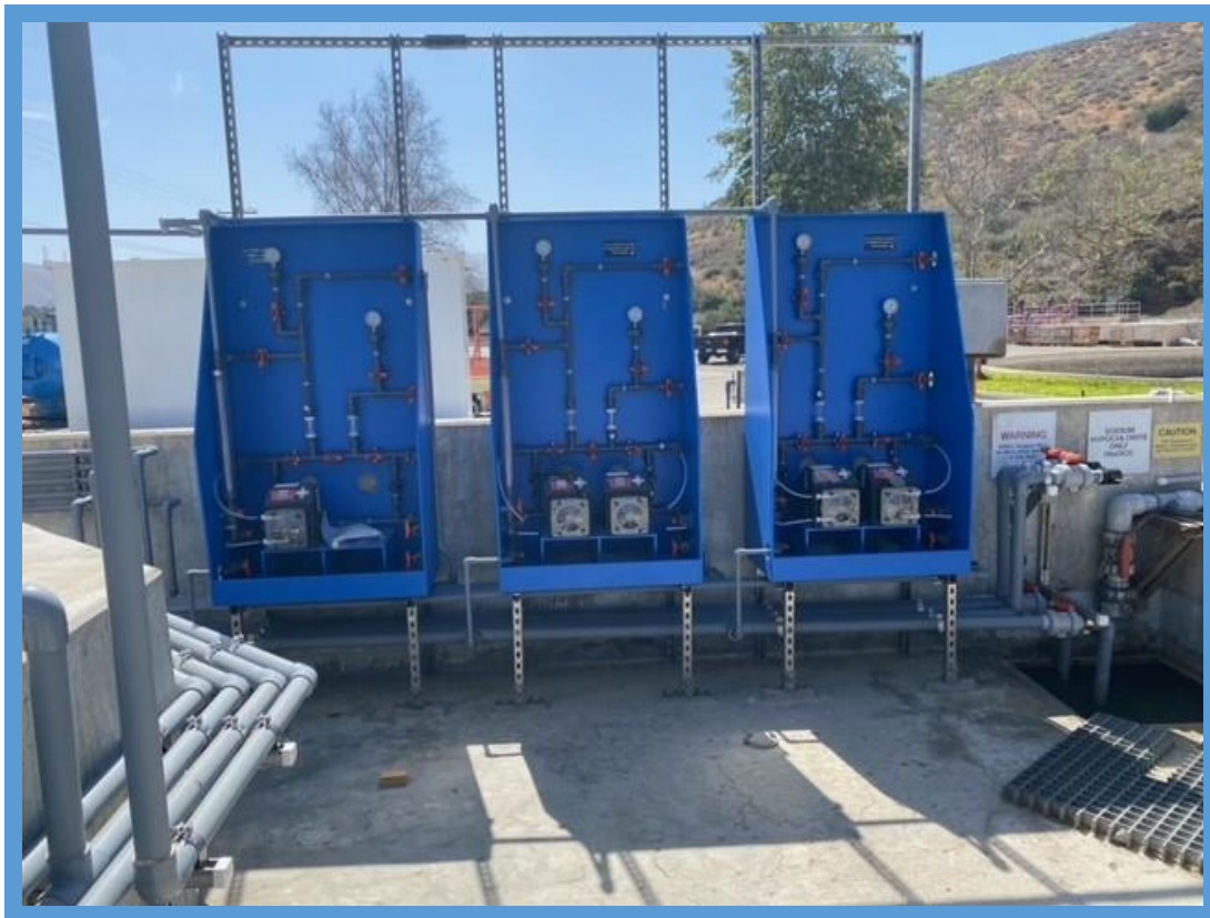
CWRF Chemical Tank and Feeder System upgrades
