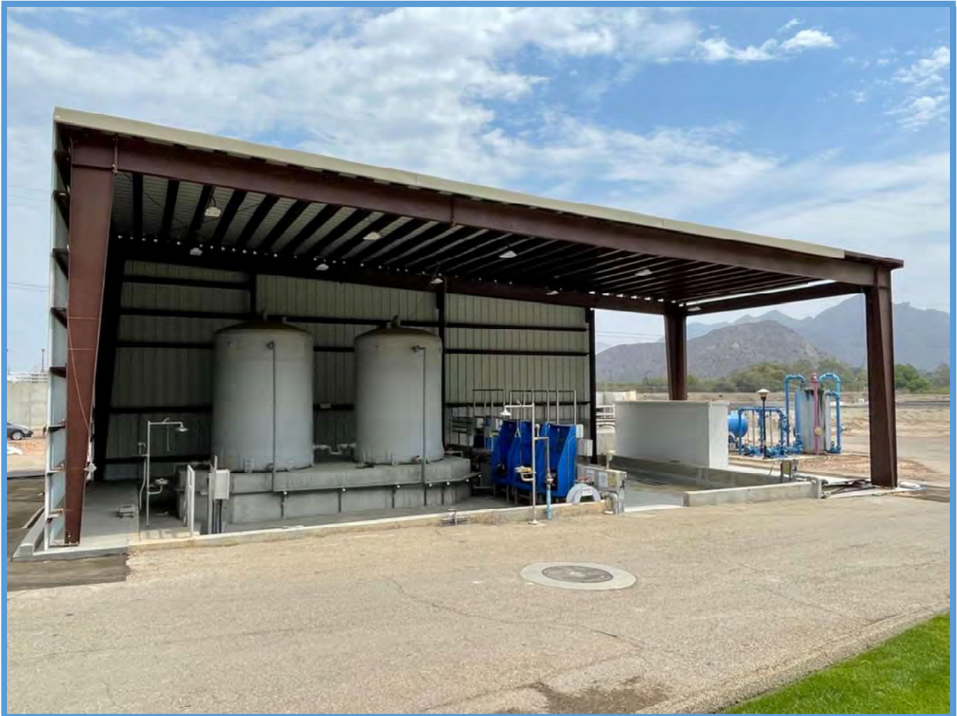
CWRF Chemical Tank and Feeder System upgrades
