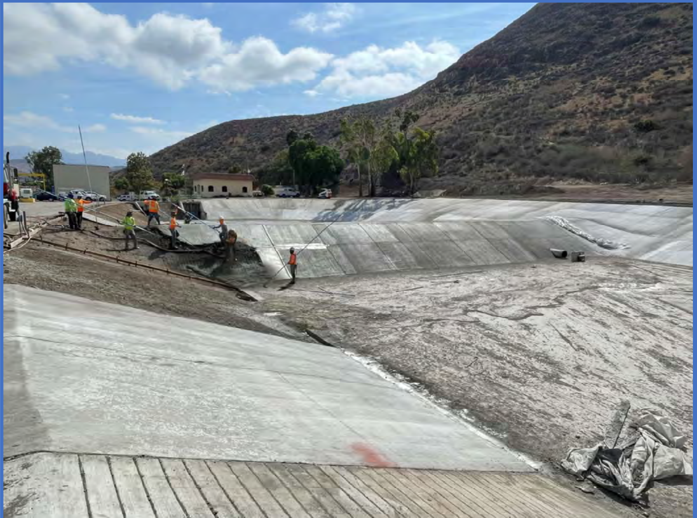
Effluent Pond Relining at the Camrosa Water Reclamation Facility
