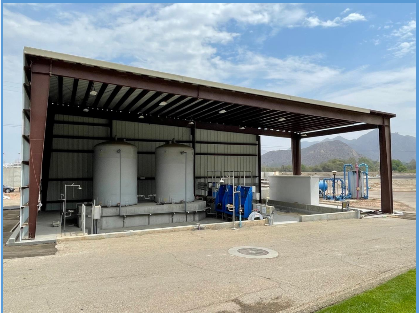
CWRF Chemical Tank and Feeder System upgrades
