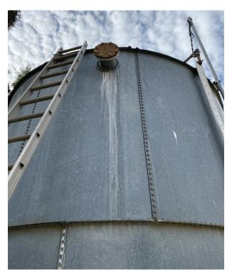
The District currently operates Well 31, the well supplies the City's 1 MGD Treatment Plant. The well site is equipped with a bolted galvanized steel tank. The tank serves to set a positive hydraulic gradient upstream of the pressure reducing valve supplying the Treatment Plant. The City planned to replace the old and corroded tank.
