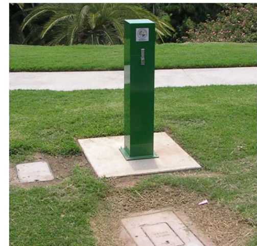
Typical Water Sampling Station
