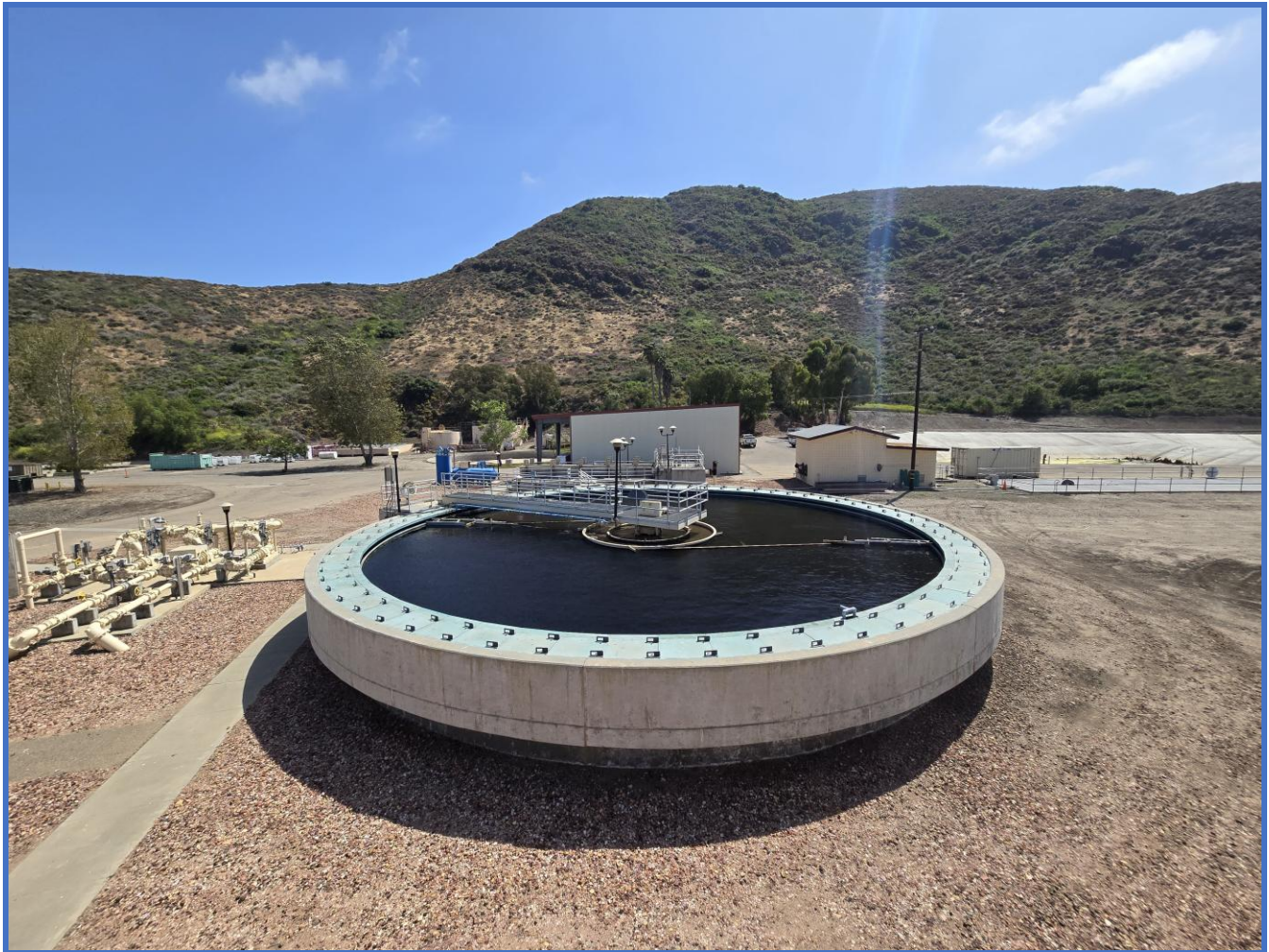
Camrosa Wastewater Reclamation Facility Clarifier
