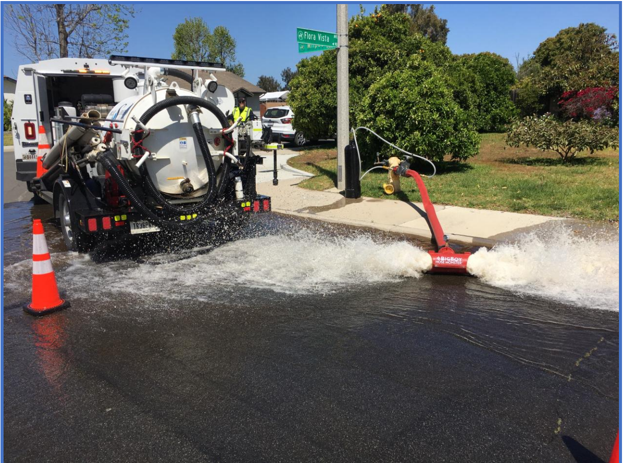
Unidirectional Flushing
