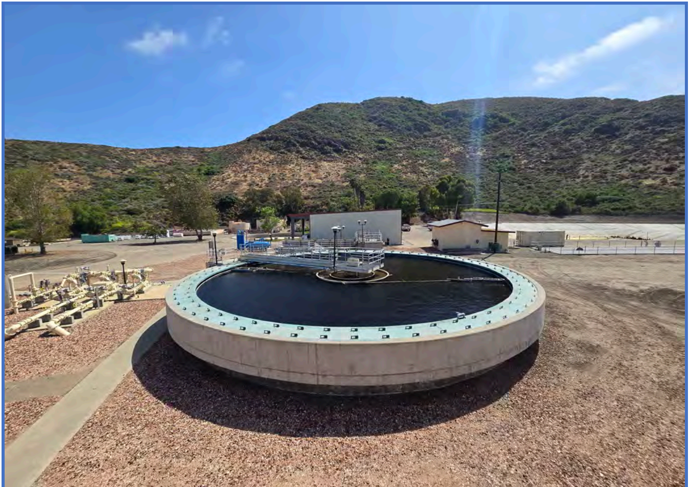
Camrosa Wastewater Reclamation Facility Clarifier
