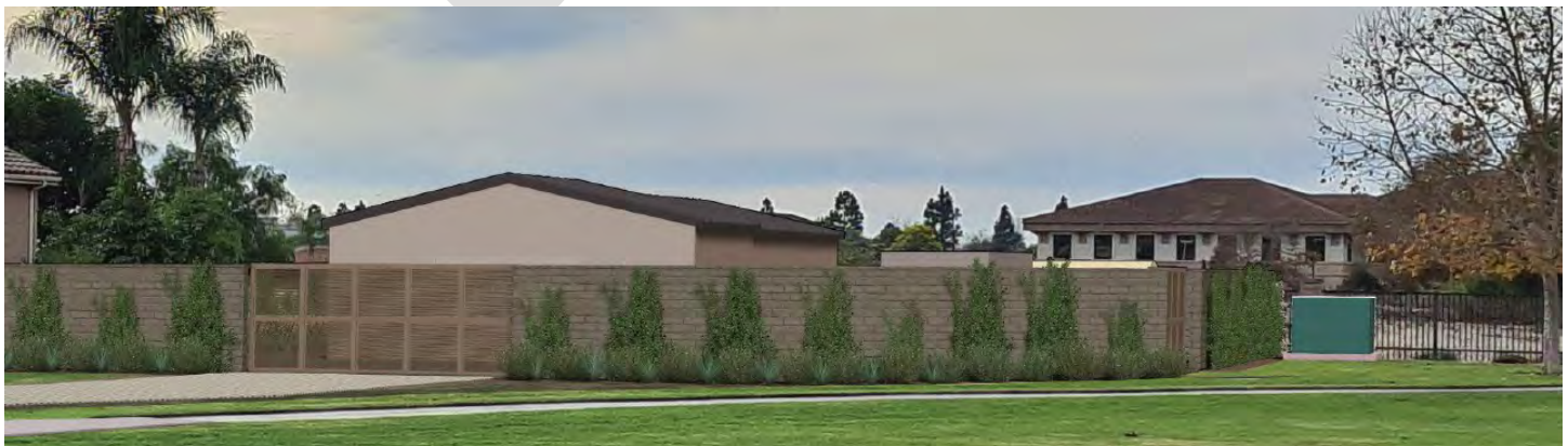
Valencia Well Preliminary Design - Completed in FY 2025-26
