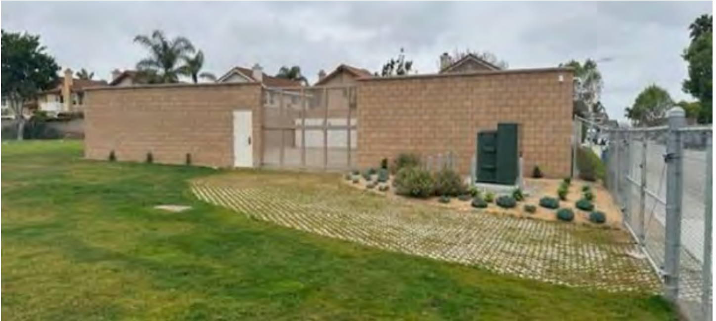
Lynnwood Well in Woodcreek Park
