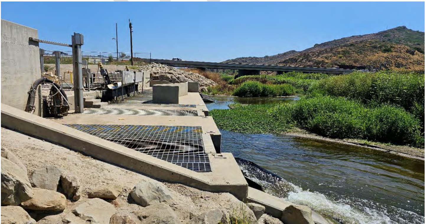
Conejo Creek Diversion
