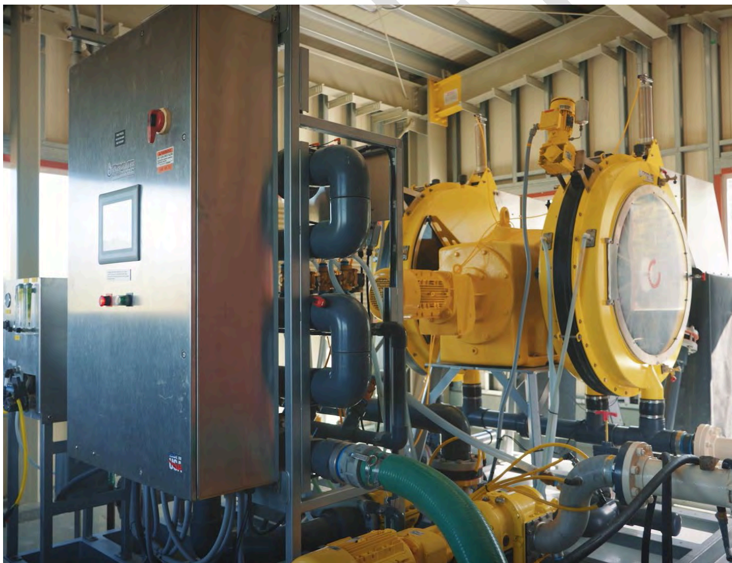
Wastewater De-Watering Press - Construction Completed in FY 2025-26
