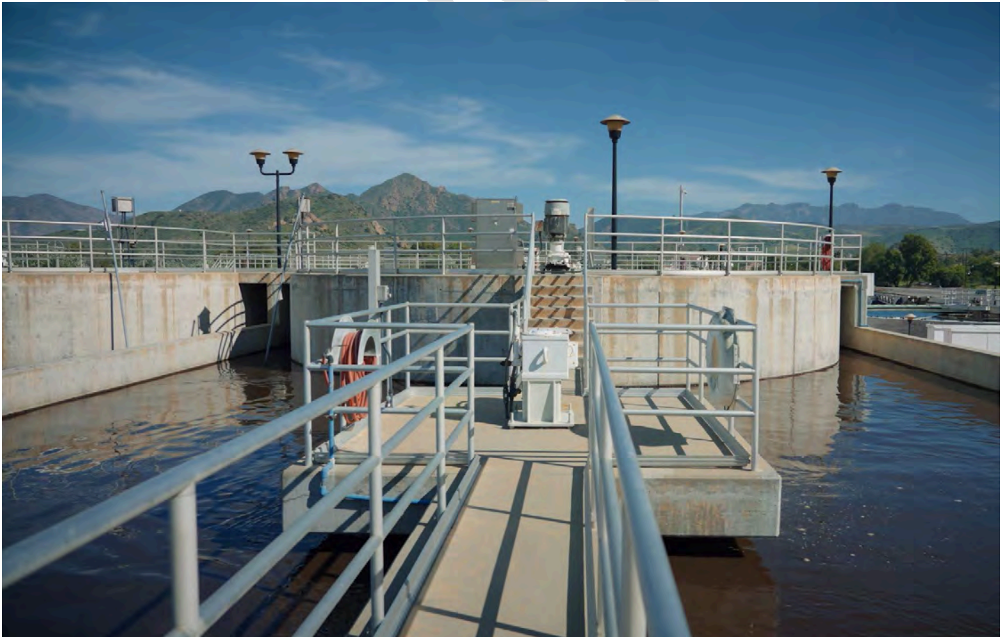
Camrosa Wastewater Reclamation Facility
