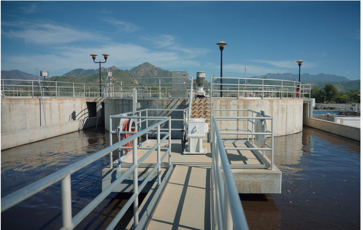
Camrosa Wastewater Reclamation Facility (CWRf)
