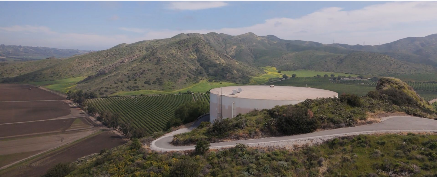
Zone 1 Storage Reservoir
