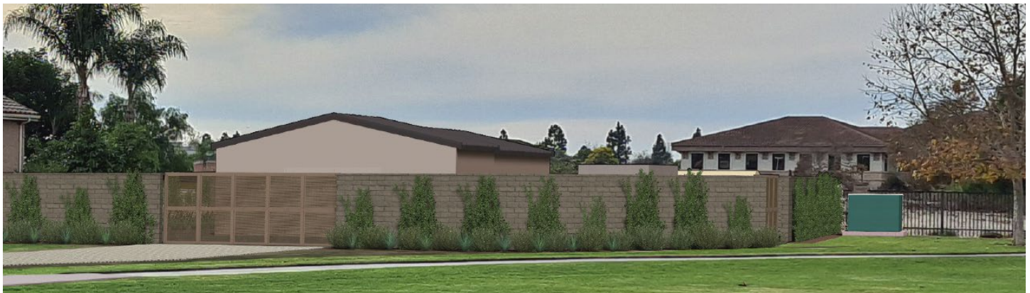
Valencia Well Preliminary Design - Completed in FY 2025-26
