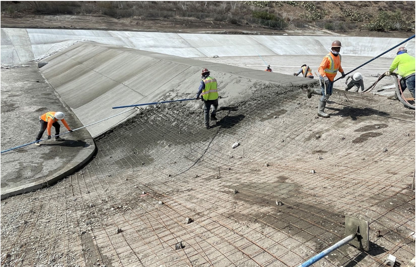
Effluent Pond Improvements at the Camrosa Water Reclamation Facility (CWRP)
