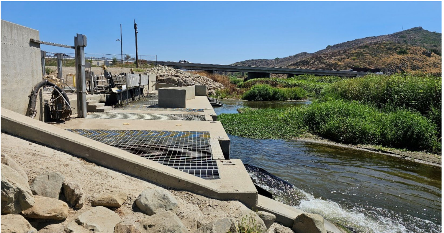
Conejo Creek Diversion
