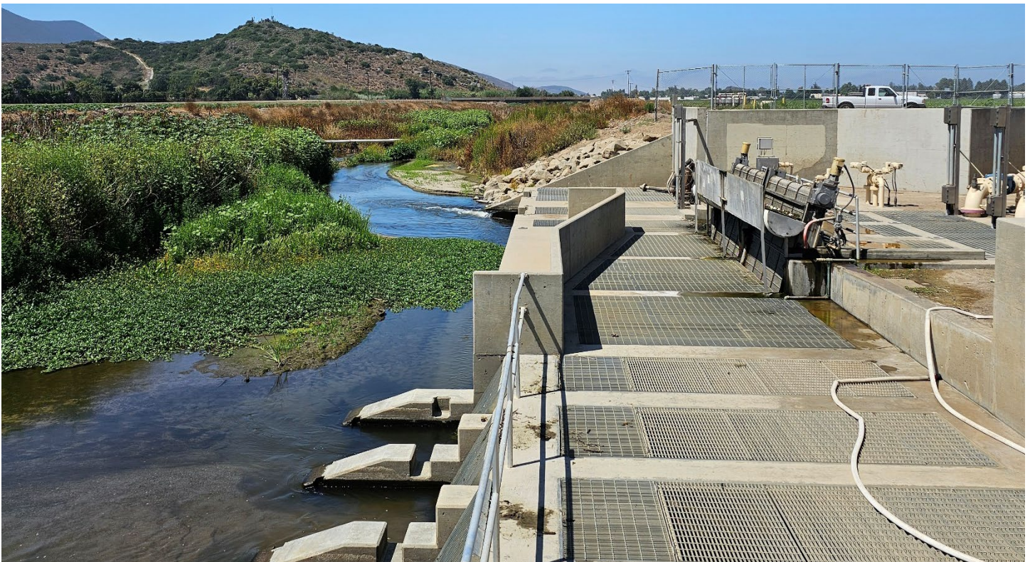
Conejo Creek Diversion
