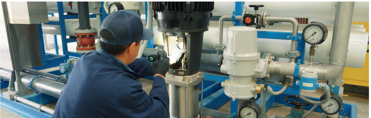
Pump Maintenance Performed by Camrosa Staff
