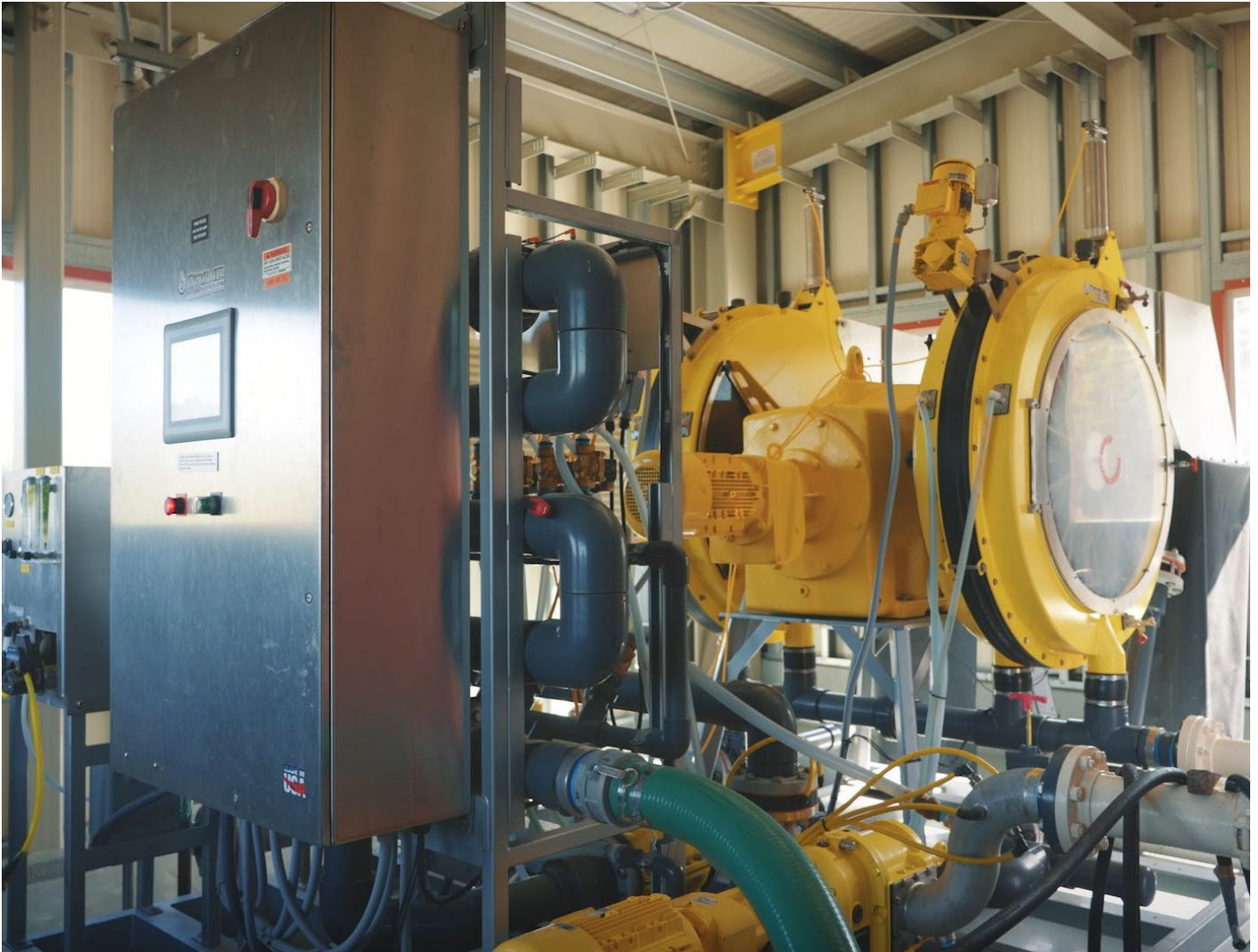
Wastewater De-Watering Press - Construction Completed in FY 2025-26
