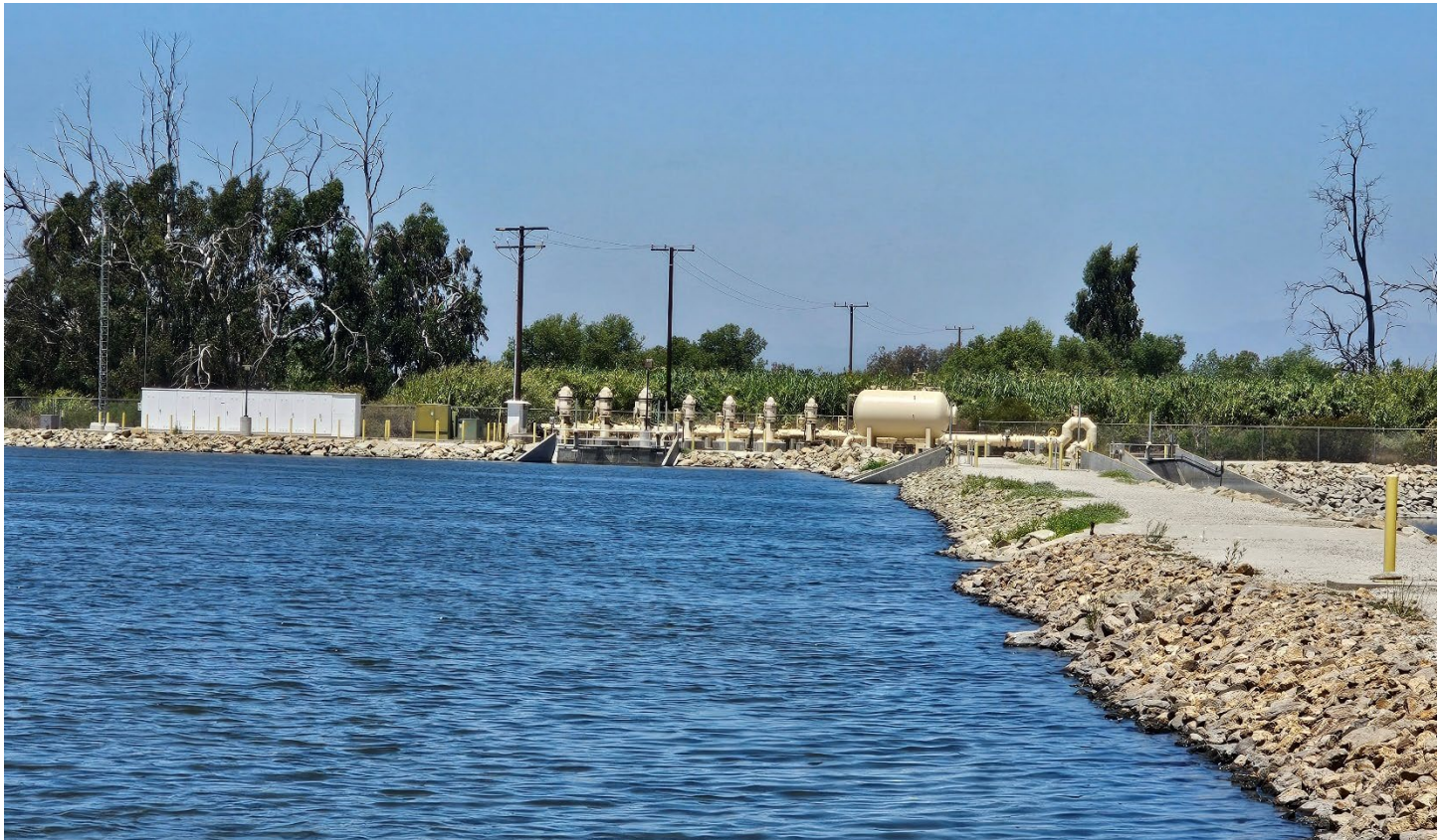
Non-Potable Storage Ponds & Pump Station
