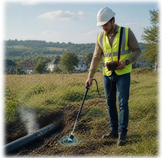
Acoustic Leak Detection
