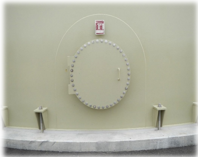
Tank Rehabilitation Completed
