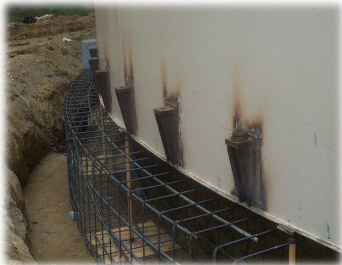
Tank Rehabilitation in Process
